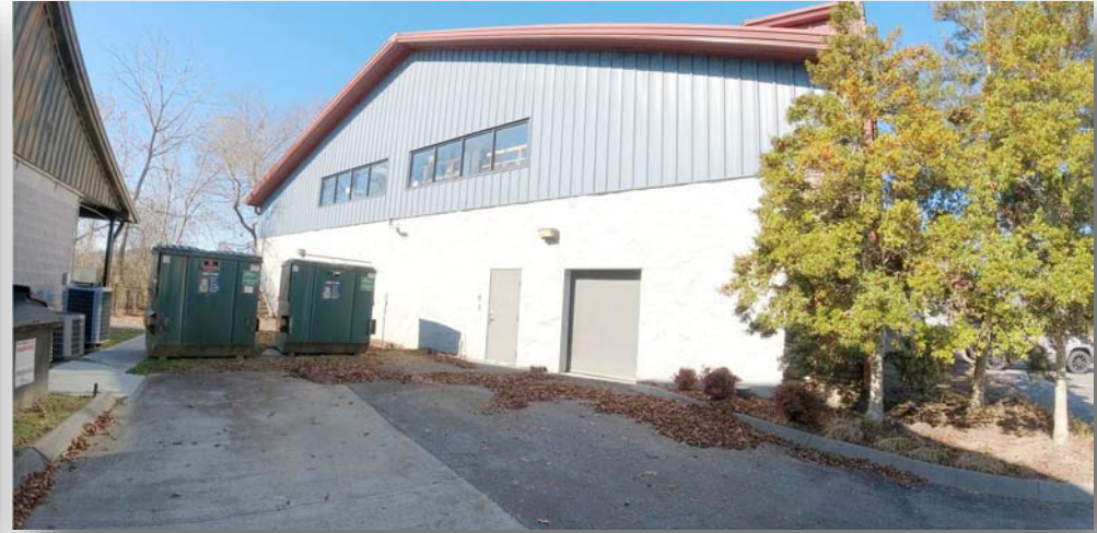
South End of Building
