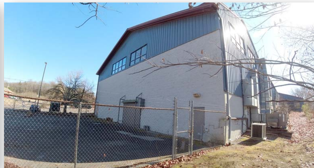
North End of Building Lower Level Entrance
