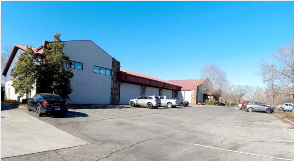
South End of Building
